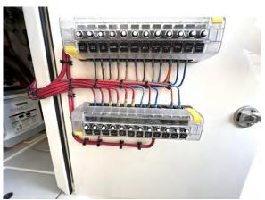
Figure 58 - DC Push to Reset Load Breakers.
