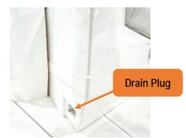
Figure 88 -Drain Plug Installed On The Sides Of Sliding Cooler.
