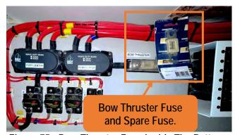
Figure 75 - Bow Thruster Fuse Inside The Battery Hatch In The Console.
