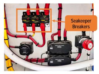
Figure 56- -Seakeeper Breakers below the Console Stairs.
