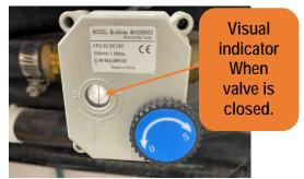
Figure 21 – motorized ball valve inside the auxiliary machinery space.
