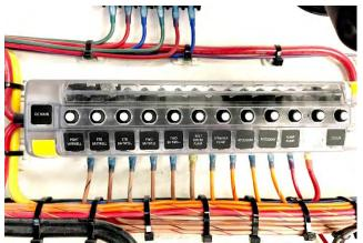
Figure 64 - DC Push to Reset Load Breakers.
