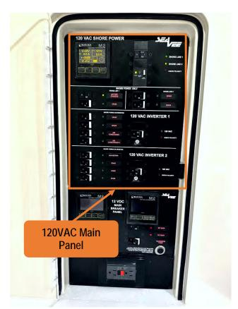
Figure 70 - 120VAC Main Distribution Panel With Shore Power Control Inside The Console.
