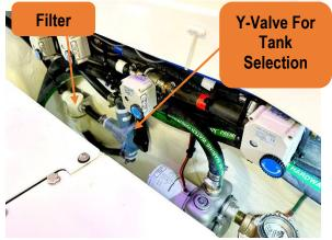
Figure 42 – Fresh Water Pump Filter Inside The Storage/Seakeeper Space.
