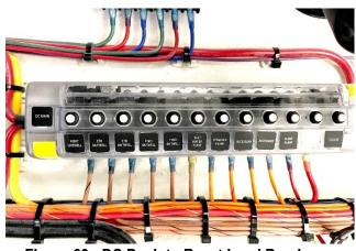
Figure 63 - DC Push to Reset Load Breakers.
