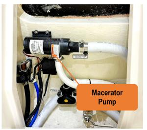
Figure 48 – Macerator Pump Access Hatch Behind Cabin Stairs.
