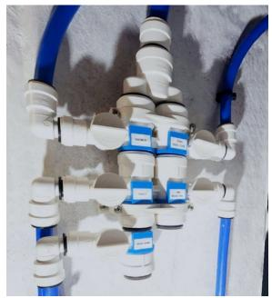
Figure 41 - Manifold Distribution.
