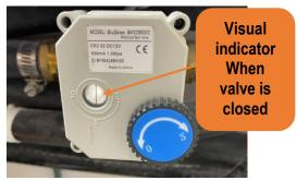
Figure 19 – motorized ball valve inside the auxiliary machinery space.
