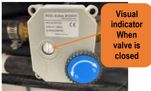
Figure 21 – motorized ball valve inside the auxiliary machinery space.
