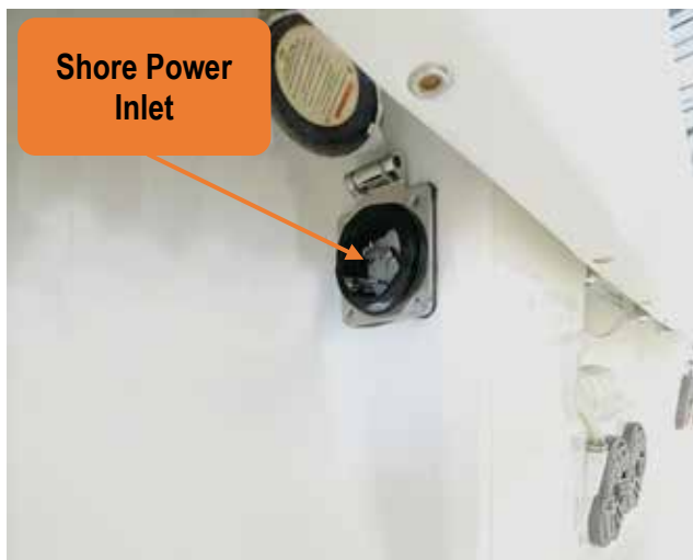
Figure 71 - shore power inlet at the starboard middle column.
