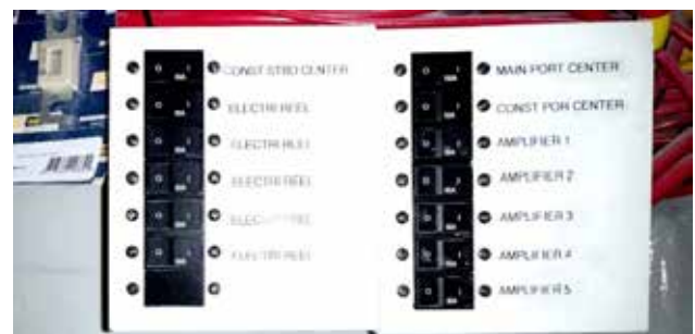
Figure 67 - 50-amp DC breakers inside the battery hatch in the cabin.
