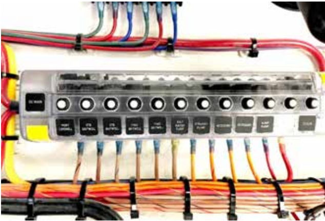
Figure 63 - dc main breakers.
