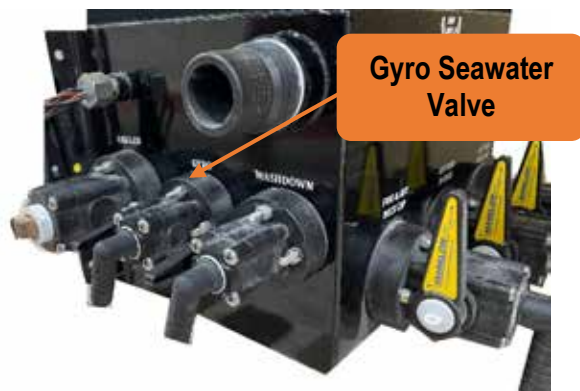
Figure 54 - gyro seawater valve at the forward face of the starboard seakeeper.
