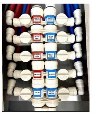
Figure 41 - manifold distribution.
